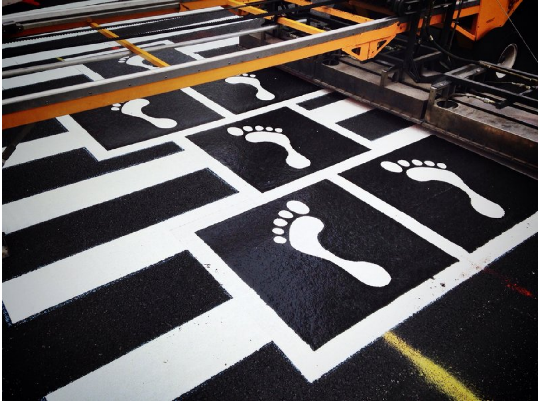
One section of the hopscotch crosswalk being installed.
